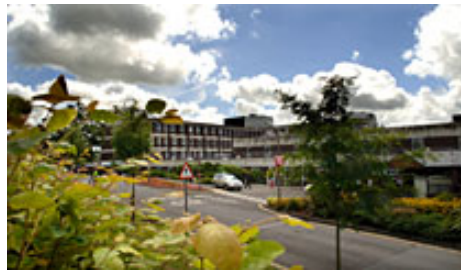
North Devon District Hospital
