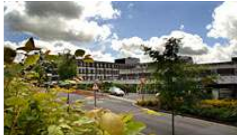
North Devon District Hospital
